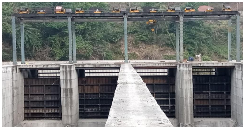
COMPLETE VIEW OF DESILTING BASIN INLET SERVICE, STOPLOG AND TRASH RACK
