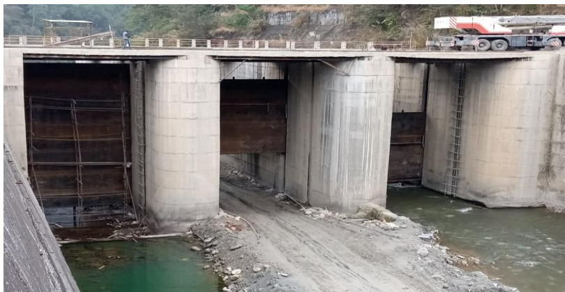
COMPLETE VIEW OF BARRAGE SERVICE, UNDER-SLUCICE GATE
