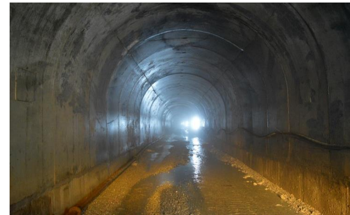
HEAD RACE TUNNEL COMPLETED
